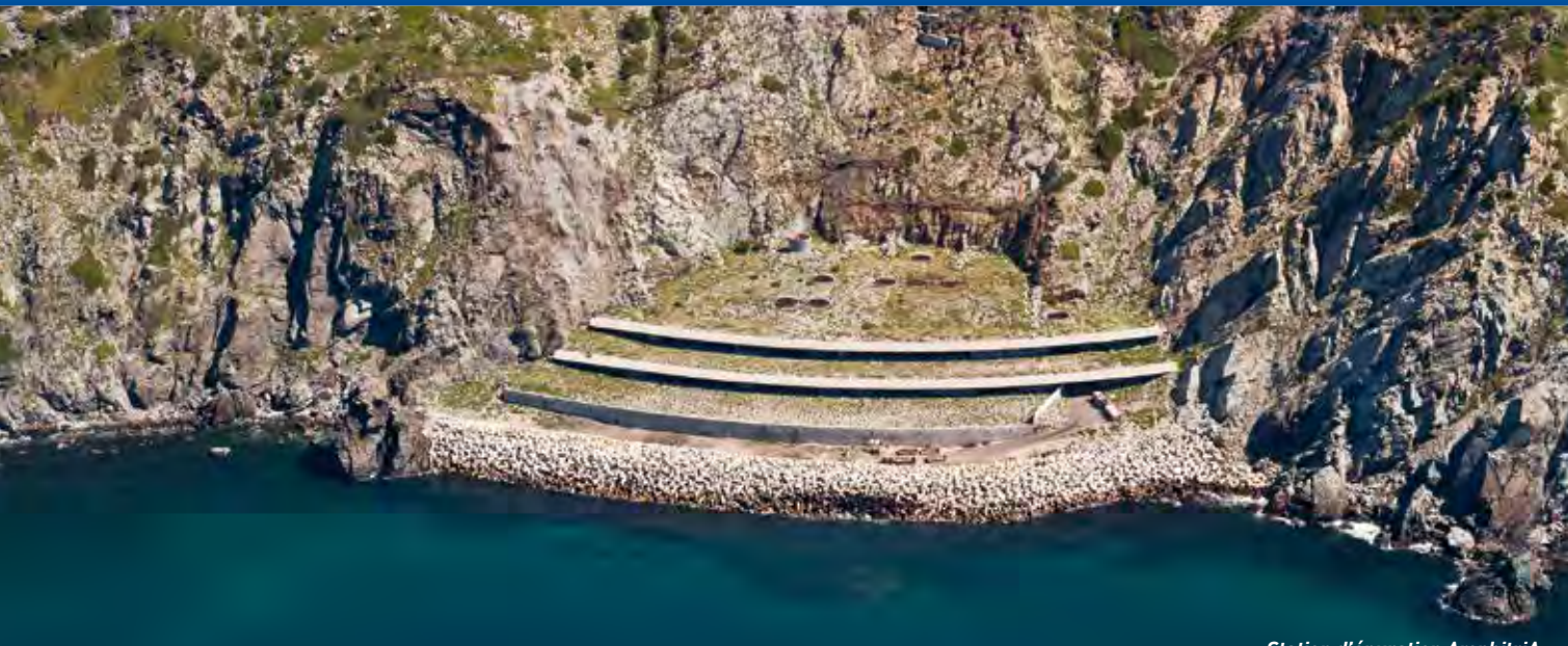
Station d'épuration AmphitriA
